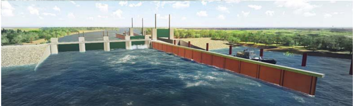
Figure 3. Sluice and ship lock with 4 gates (Source: Royal HaskoningDHV, 2020)
